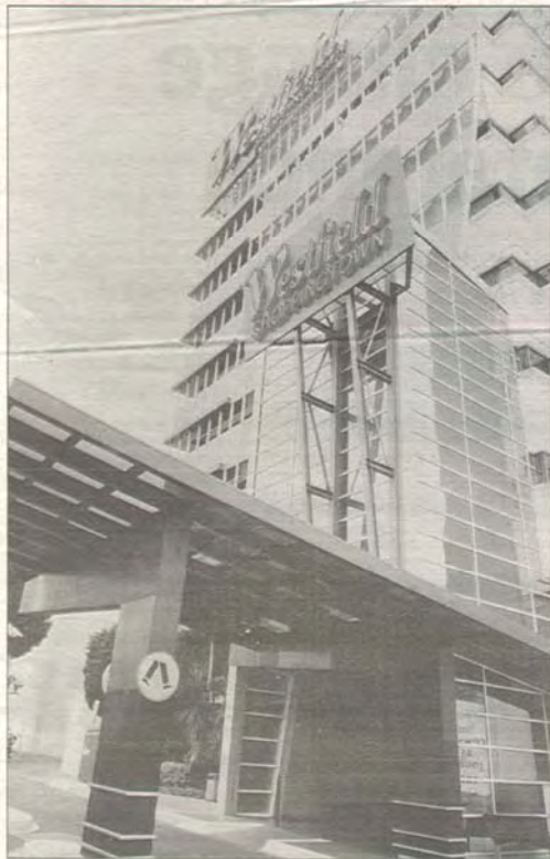
To the point: the angled beams at the Doncaster Shoppingtown. 020MK300
